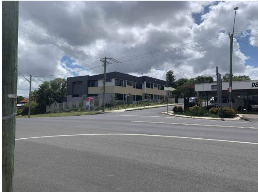
115 CENTRE STREET - EXISTING RESIDENTIAL FLAT BUILDING
